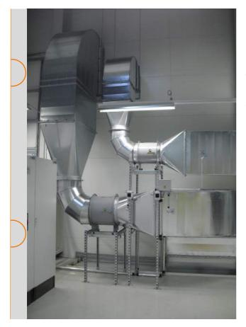
Duct elements are produced with rolled sheet angle profile and corner profile. The widths of angle profiles are 20 or 30 mm. Sealing material of air duct elements Nr. 4209/ OF/0602 is used. It is fiber reinforced waterbased duct sealant, thermostabile up to 1000 °C, one-component, solvent-free.
