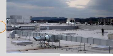
The rectangular air ducts and fittings manufactured by Radel & Hahn Zrt. made of galvanized steel sheet with a rectangular cross-section, according to the Austrian standard ÖNORM M7615, are made for ventilation systems and can be used for various purposes, taking into account the required air velocity, pressure difference and airtightness.
